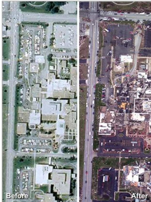
St. John's Hospital, Joplin, MO, before and after the EF5 tornado on May 21, 2011. The hospital sustained a direct hit by the tornado. Photo credit: NOAA.
